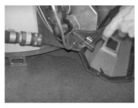
Step 3: Disconnect Pilot Fitting from Burner Box
